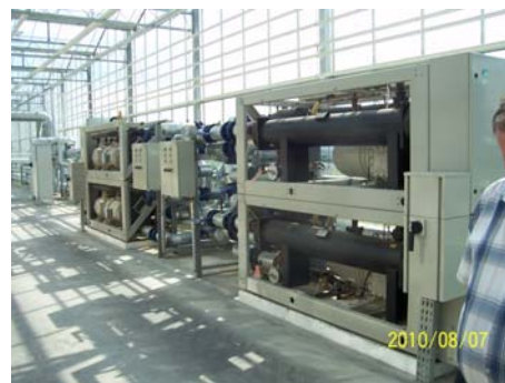
Figure 13: Heat pumps Daikin EWWD 440MBYN at the Greenhouse Complex “Berestye”.
